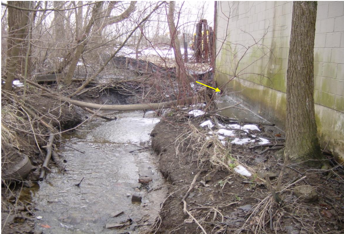
Meandering, unstable channel undercutting building
