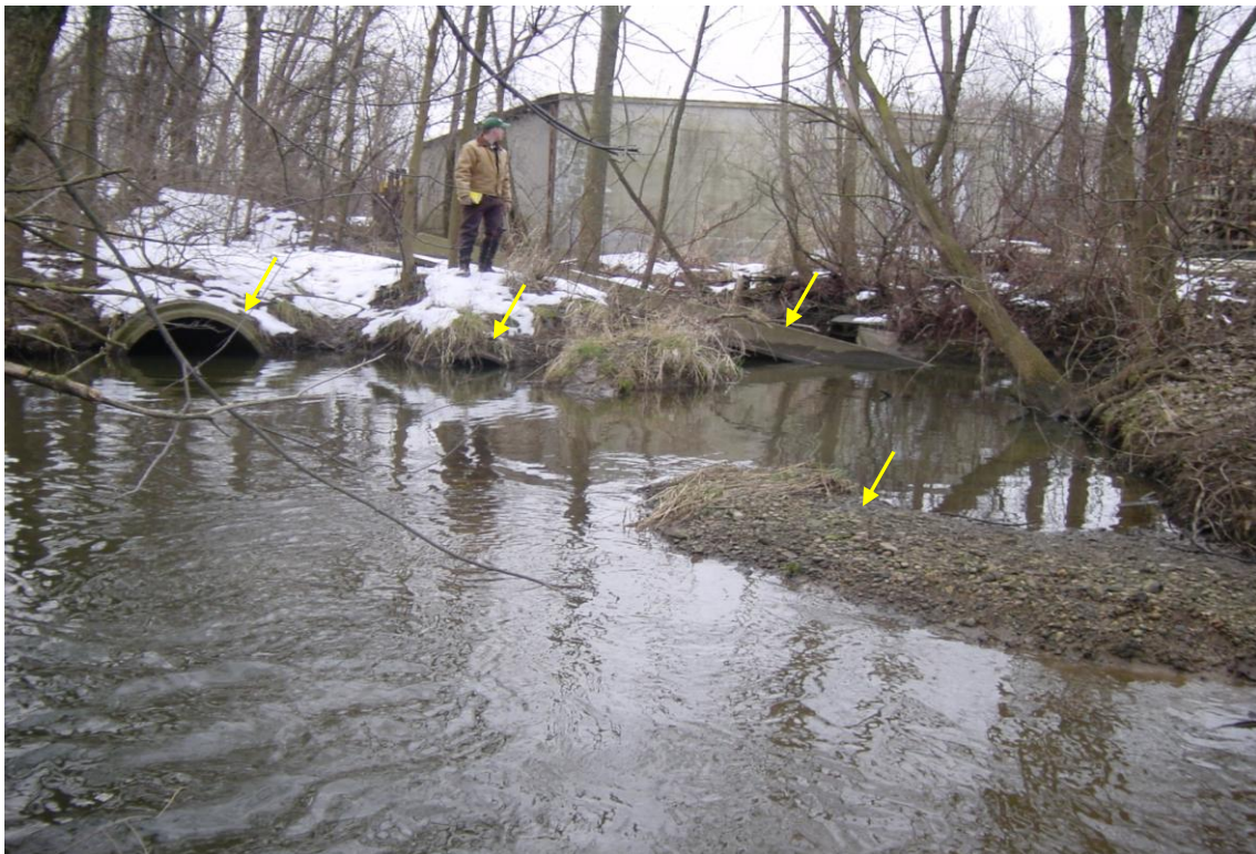
Sediment bars, blockages and failed culverts
