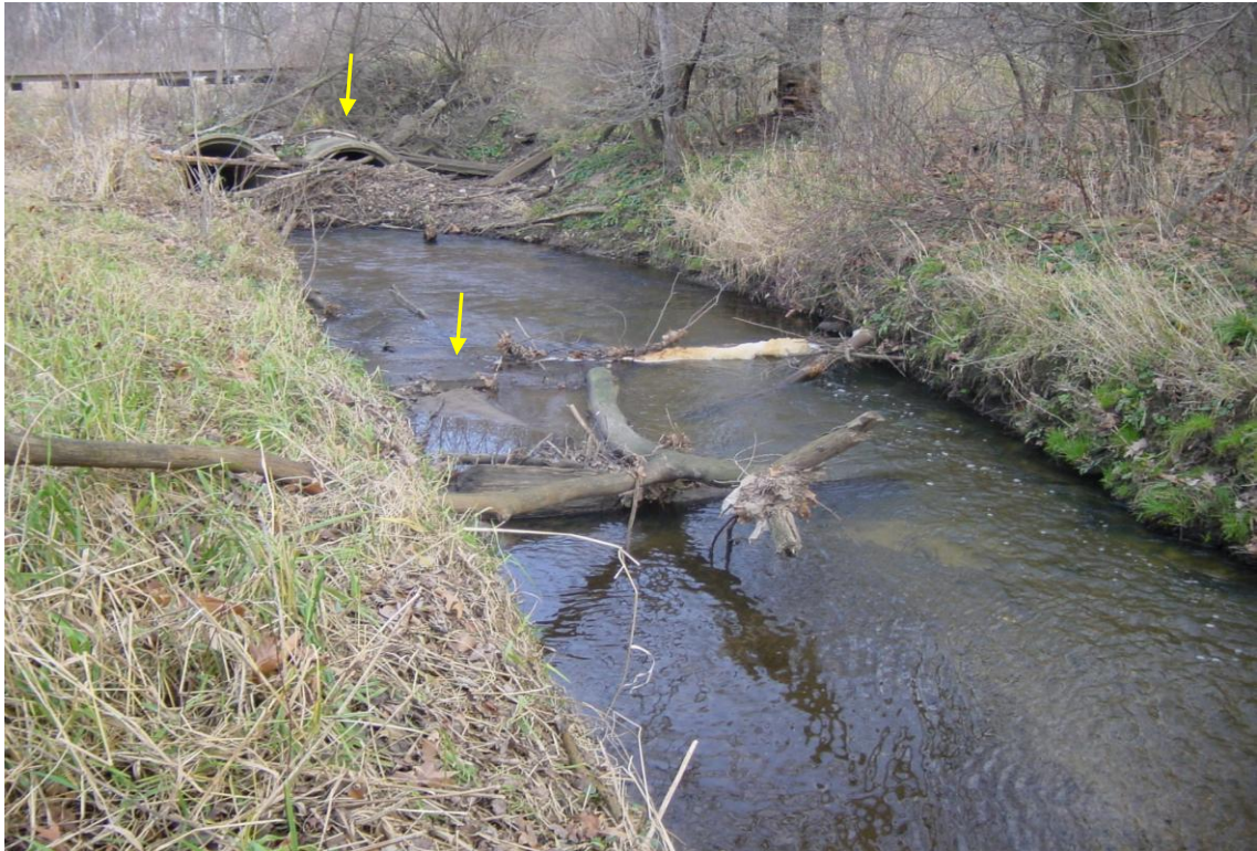
Blockages upstream end of twin culverts; sedimentation
