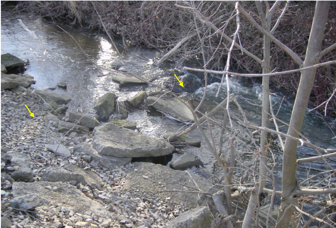
Failed stabilization efforts; excessive grade
