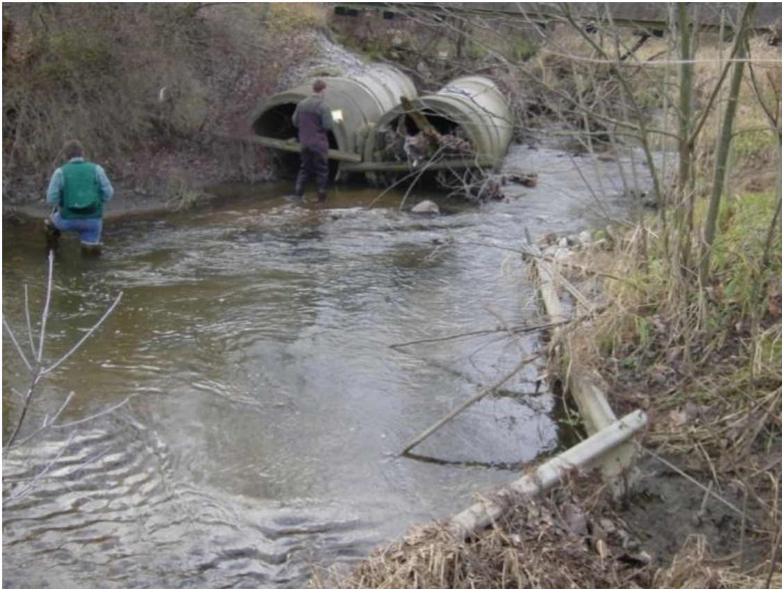
Failed culverts; bank erosion; blockages; sedimentation
