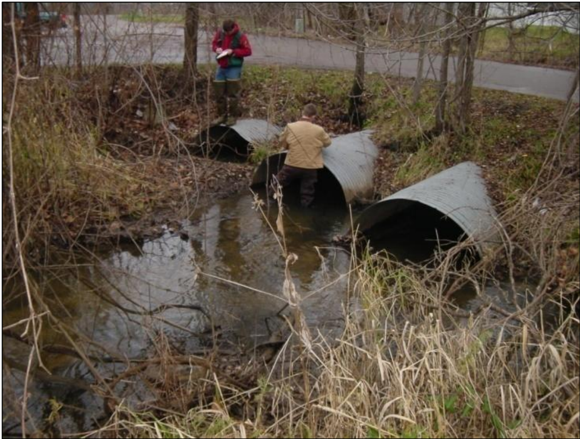
Plugged culvert
