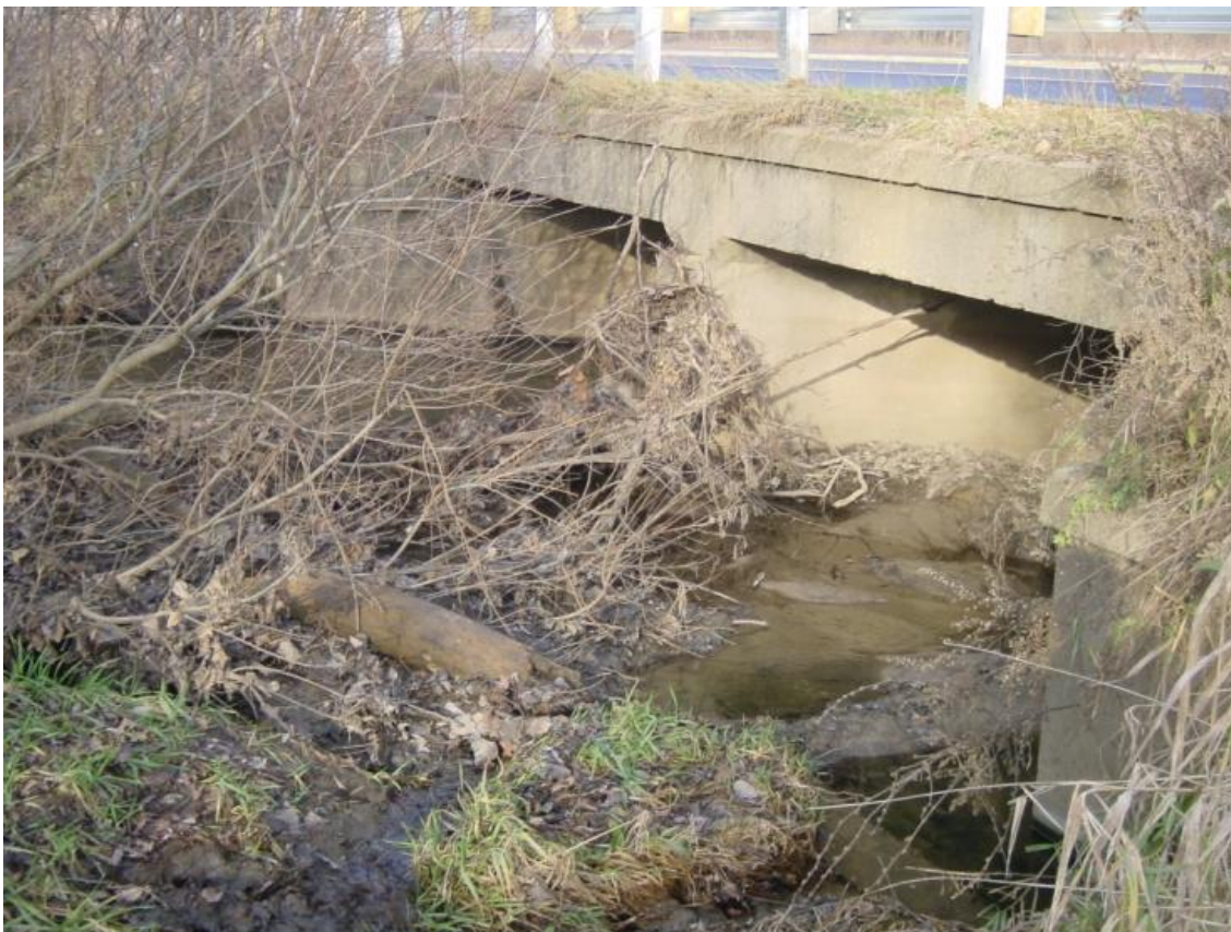
Sedimentation upstream of failed twin culverts
