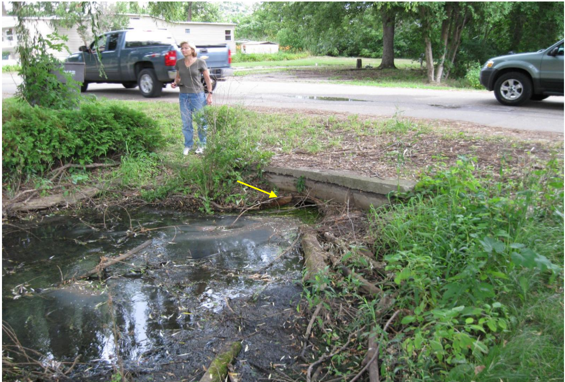
Plugged culvert; stagnant water
